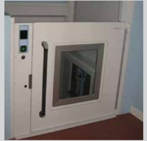
Half Height Gate at Upper Level
